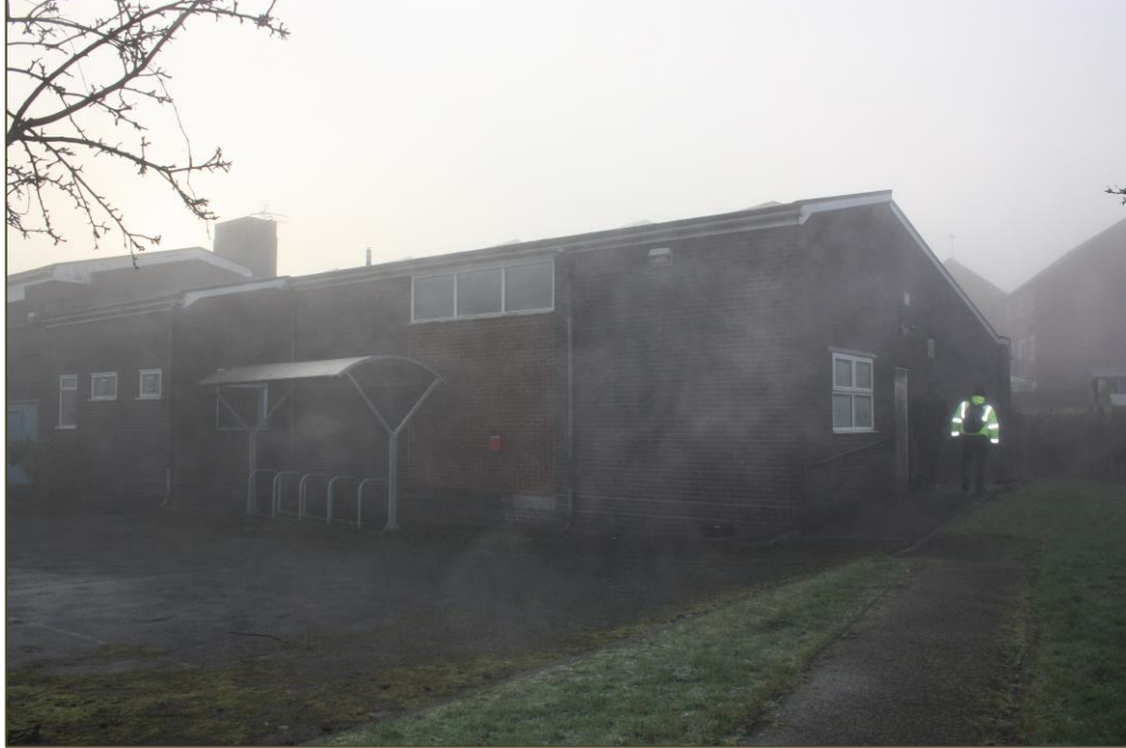
Plate 3: An image showing the northern and eastern elevations on the structure.
