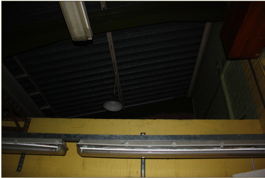
Plate 7: A photograph showing the internal corrugated steel roof.
