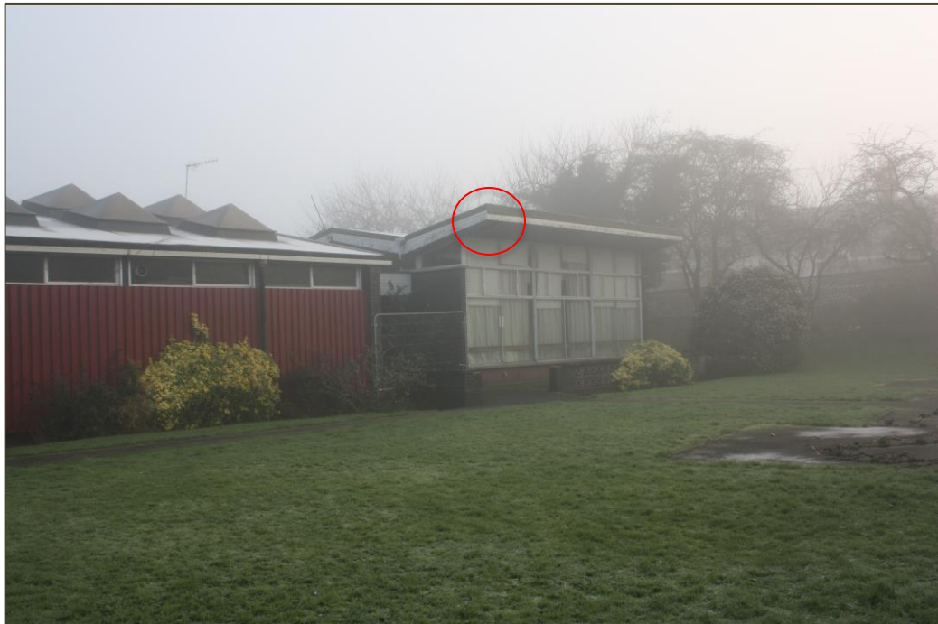
Plate 4: An image of the southern elevation of the building (Hotspot Area 2, is indicated by the red circle)
